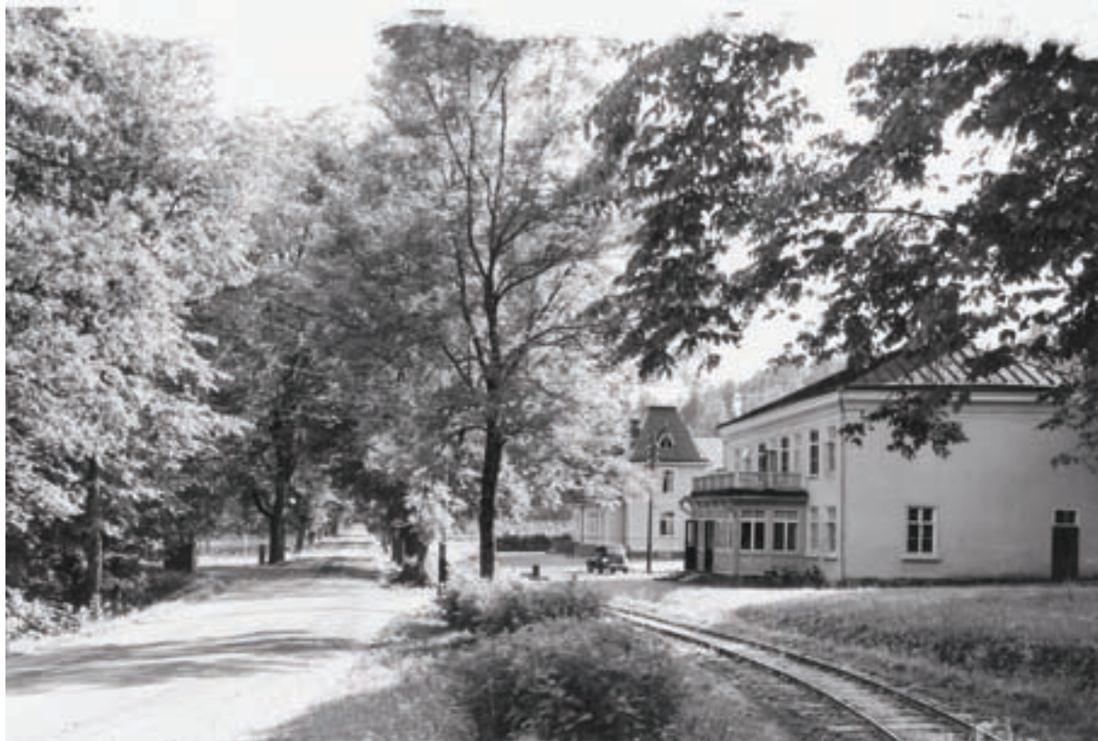
The Wårdshuset, the inn, built in 1836, in front of which the rails of the narrow-gauge track can still be seen. The line was last used in 1952.
