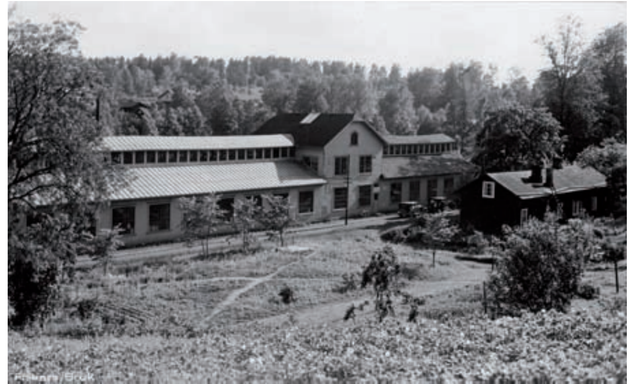
Originally built as a plow workshop in 1914, this building was extended to include new factory space in the 1970s. Today, it houses workshops and offices.
