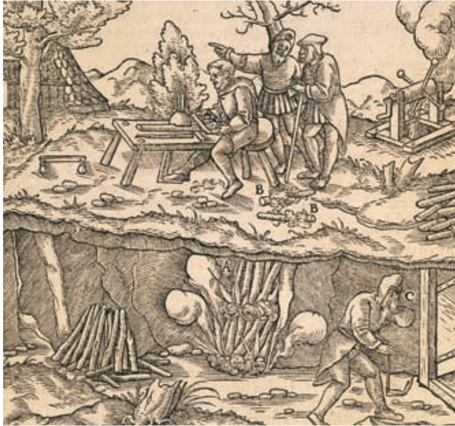
Preparing kindling and fire wood at the rock face, stages in an early method of ore extraction.
